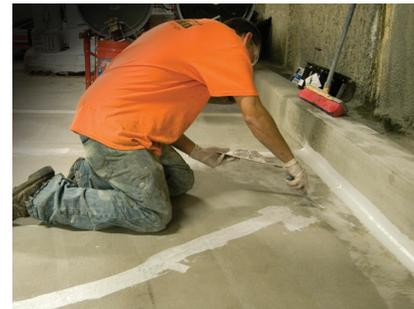
Stonhard applicator applying a crack treatment before applying Stondeck product
